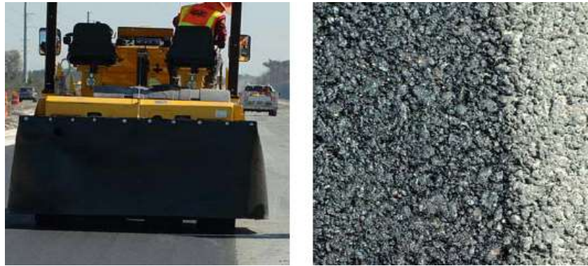
FIGURE 8. Tight longitudinal joints with no aggregate crushing
