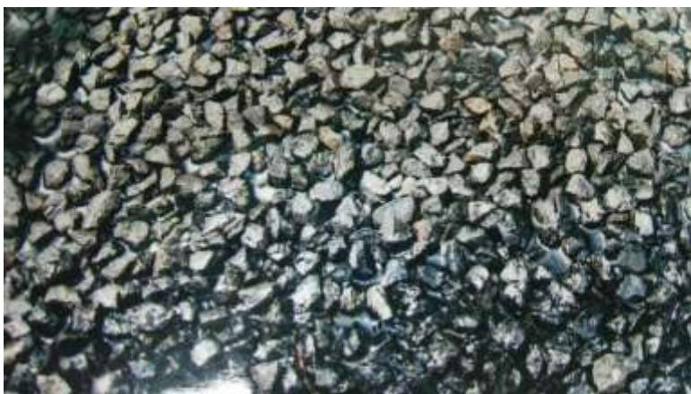
FIGURE27. Finished surface after compaction of VPT roller
