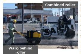
Demonstration tests of electric combined rollers and electric walk-behind rollers were conducted at actual construction sites.
