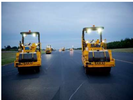
Highway paving in the U.S.
