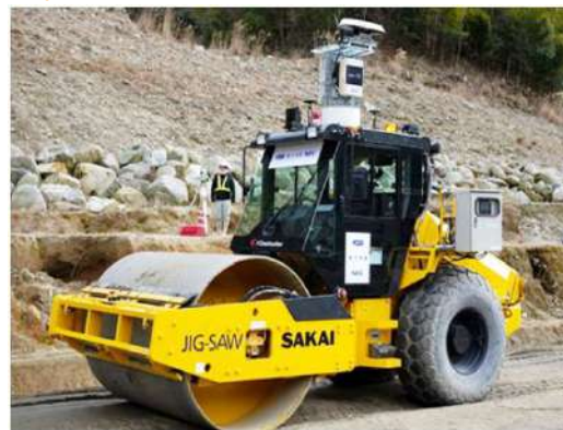
Autonomous roller- Test marketing to be completed
