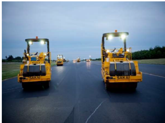
Highway paving in the U.S.
